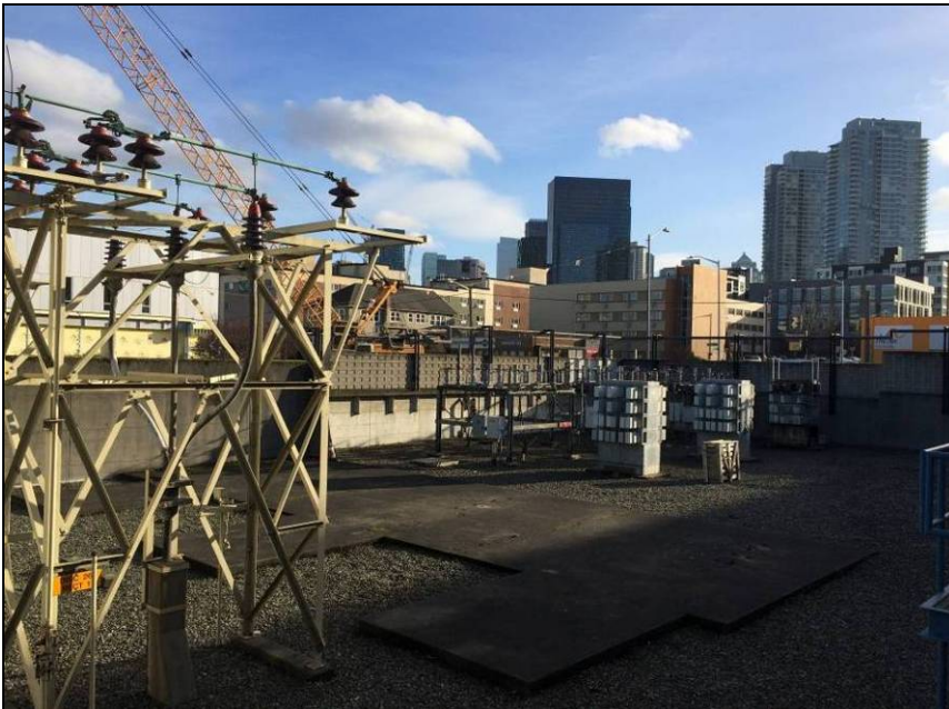
Figure 15. Below, looking southeast from the switchyard at the security walls and fencing on the perimeter east and south property lines.
