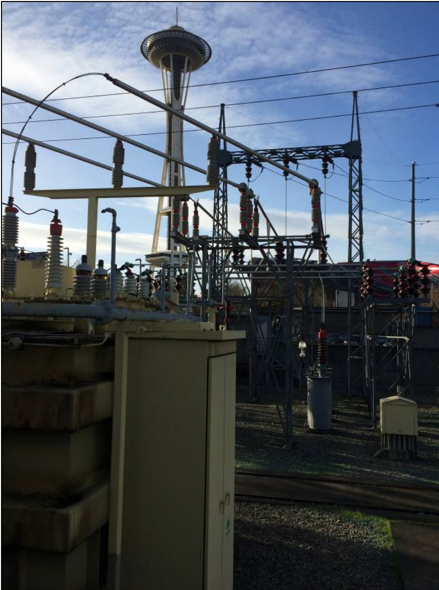
Figure 19. Above, looking west from within the switchyard at busses with insulators with the Space Needle in the background.
