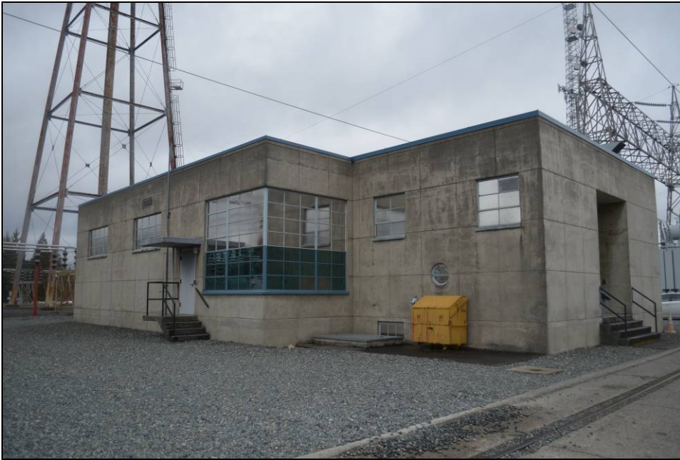
Figure 66. Above, the Bothell Substation, southeast facade of the Control Building, which was designed also by Ivan Palmaw in 1949 (Seattle City Light, DSC-0365). Note the grid pattern concrete, small circular window and larger corner window.
