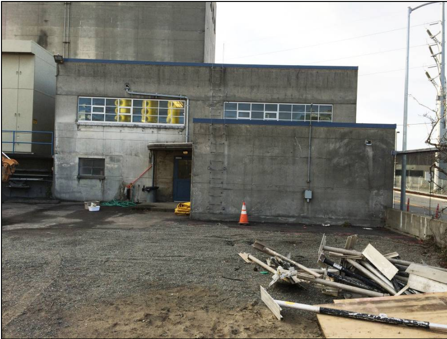
Figure 38. Below, looking west at the east facades of the Shop and Pump Room. Note the original wall-mounted steel access ladders and window openings and recently installed aluminum frame windows.
