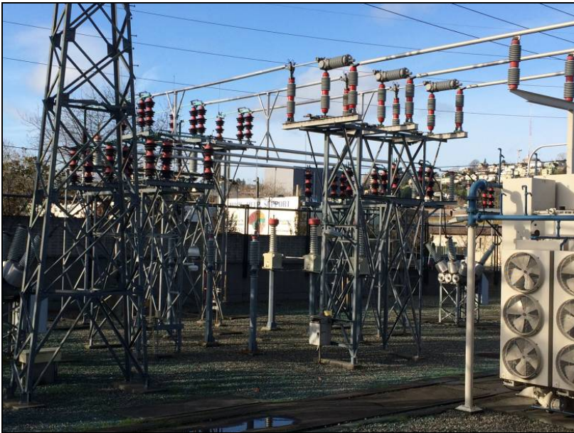
Figure 18. Below, looking southwest in the switchyard at busses and vent fans on the side of the transformers and switchgear equipment.
