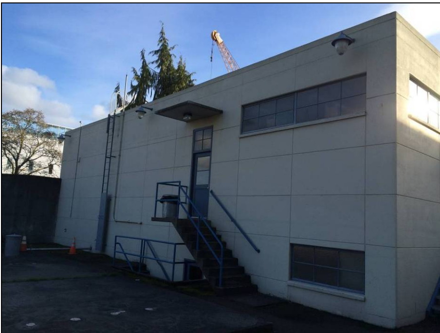
Figure 26. Below, oblique view of the Control Building's north facade.
