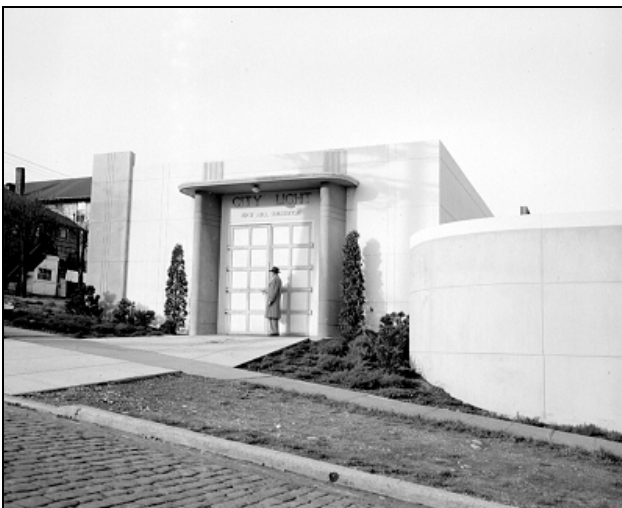
Figure 70. Left, the former First Hill Substation, with its Art Moderne style building and walls, on January 5, 1952 (demolished 1996). This property has been acquired by Seattle University (SMA, item 23345).
