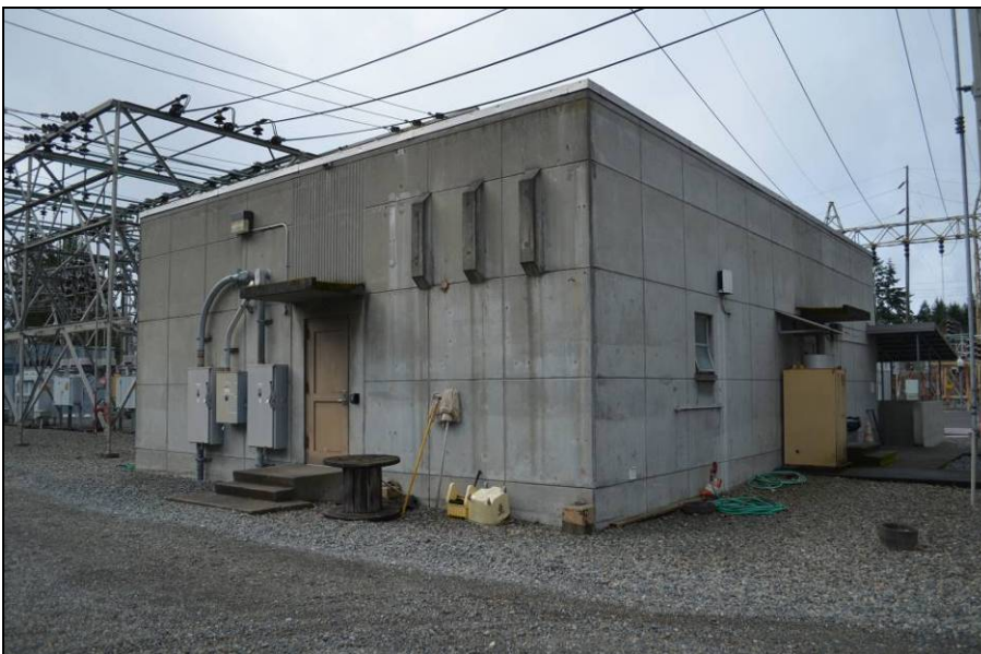
Figure 65. Below, the Shoreline Substation, northeast facade (Seattle City Light, DSC-0415).
