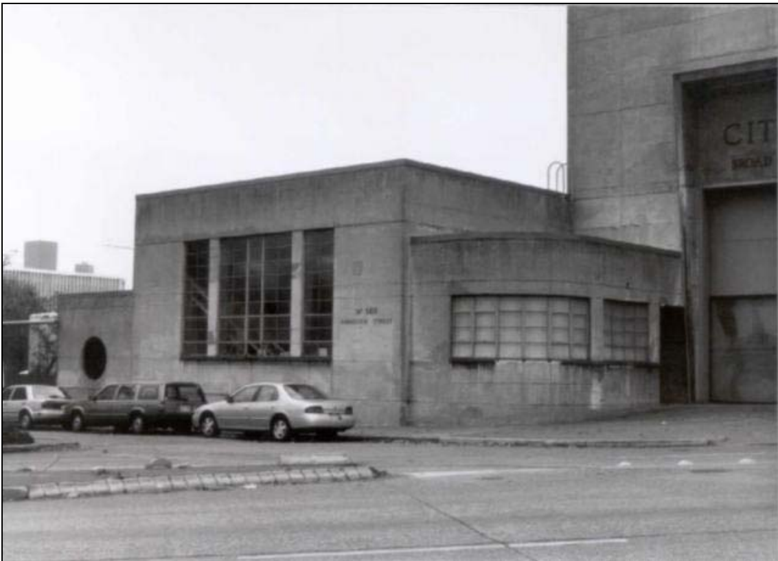
Figure 89. Below, looking southeast at the Office, Shop and Pump Room sections of the Crane Building, showing the original steel sash windows and circular window (Wickwire, DON Inventory Form, October 2000).
