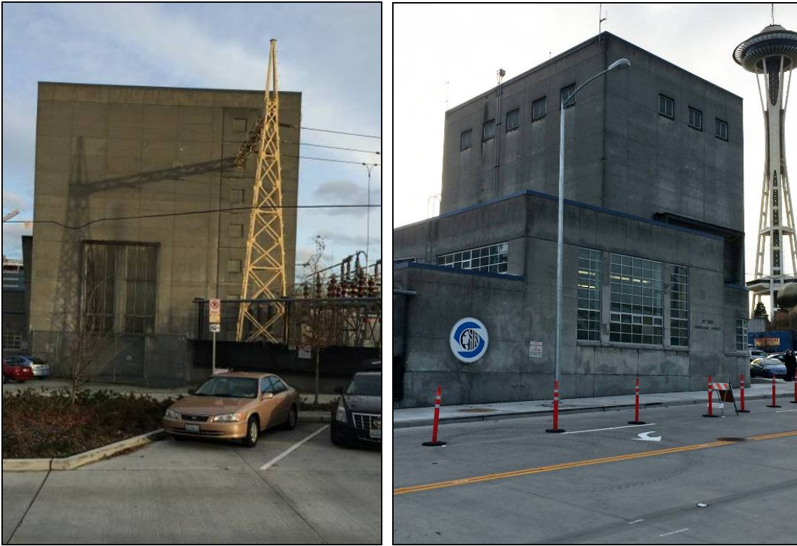
Figure 32. Above left, looking east at the lattice-tower and west facade of the Crane Tower.
