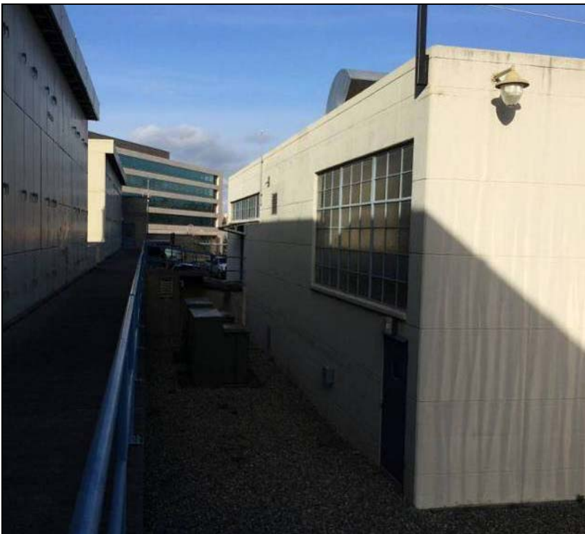
Figure 28. Below, looking north at the west corner of the Control Building and raised walkway along the east side of the switchgear equipment.
