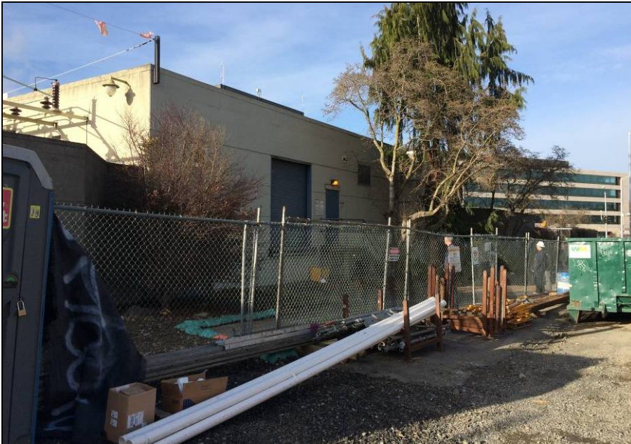
Figure 23. Above, looking northwest at the east facade and a portion of the north facade of Control Building. The fencing in the foreground is temporary.
