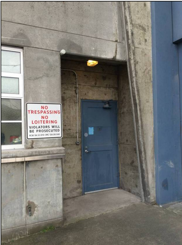
Figure 36. Left, detail view of the recessed entry and entry to the office within the Shop, west facade.
