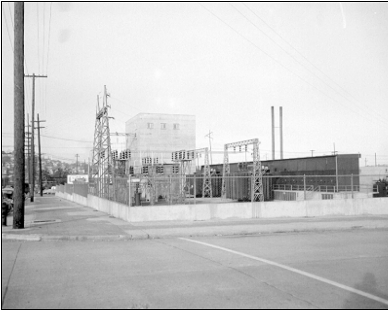
Figure 82. Above, looking northeast at the substation from the corner of 5 th Avenue N and Taylor Street in late 1951, showing original low concrete wall and woven wire fences (SMA 23341).
