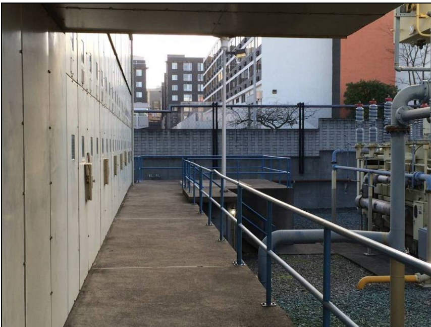
Figure 22. Below, looking south on the raised platform on the west side of the switchgear with some of the concrete block perimeter wall and fencing visible in the background.
