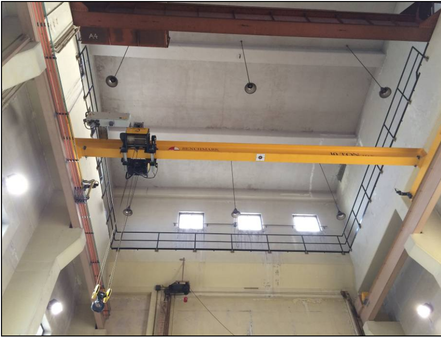
Figure 41. Above, interior of the Crane Tower, looking up at the upper south wall and the two cranes, and the catwalk around the upper portions of the east, west, and south walls.
