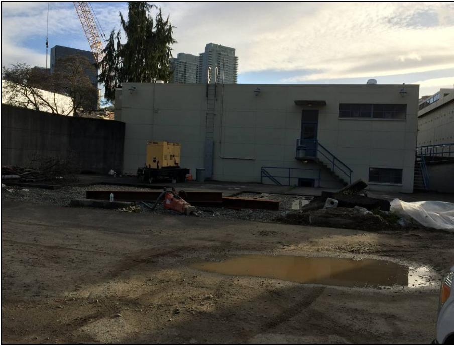
Figure 25. Above, looking south in the parking area, within the site, at the north facade of the Control Building.
