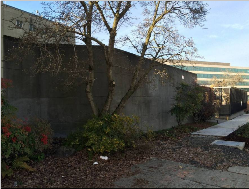
Figure 12. Above, looking northwest along the perimeter wall located to the east of the Control Building along 6 th Avenue N. Landscape materials are placed within the property setback.
