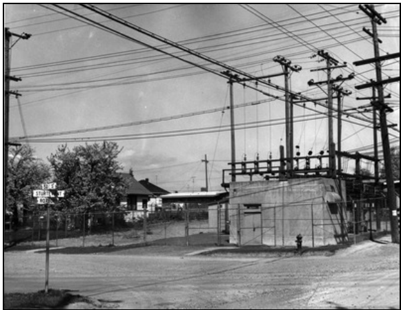
Figures 71 - 73. These photos of nearby substation illustrate their relative consistency as switchyard design became based more on manufactured components rather than customized or shop-built elements, such as transformers. Above left, the Bothell Substation bus fork, October 7, 1964 (SMA 168190), and right, the Duwamish Substation on May 23, 1955 (SMA 172931). Below, the Roxbury Substation in 1956 (SMA 173647).
