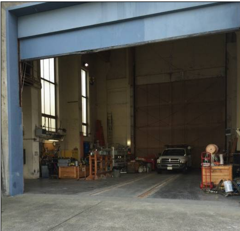
Figure 40. Below, looking south through the main vehicle entry into the interior of the Crane Tower. Portions of the original rail track remain in the floor slab.
