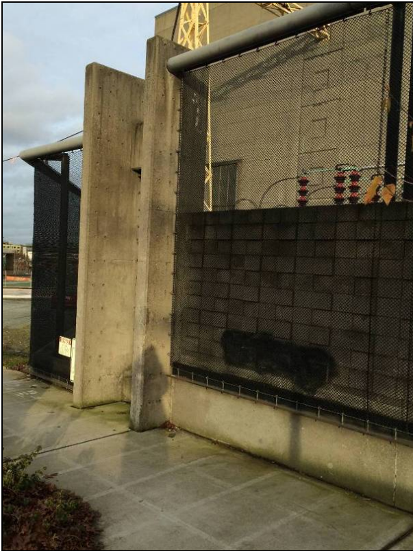
Figure 14. Above, looking northeast on 5 th Avenue N at the concrete fin walls and metal pipe and steel chain link fence near the northwest corner of the site.
