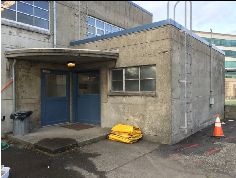
Figure 39. Above, detail view of the southeast canopy and entry doors to the Shop and Pump Room (east and north facades).
