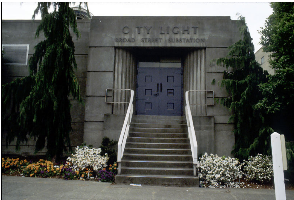
Figure 91. Below, primary entry, east façade of the Control Building, December 2001 (SMA 123776). The building's concrete perimeter walls were not painted at this time.
