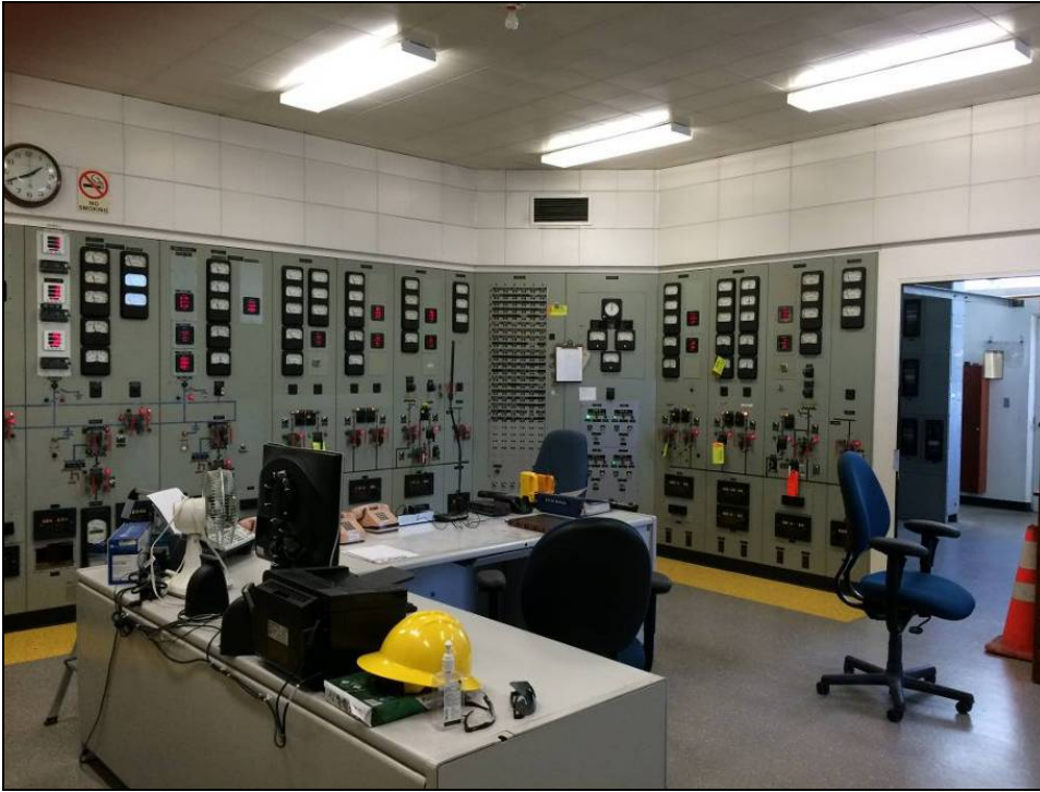
Figure 29. Above, the first floor Control Room in the Control Building.
