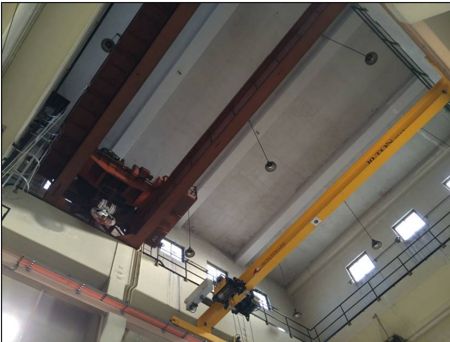
Figure 42. Below, interior of the Crane Tower, looking up toward the southeast corner at the cranes.
