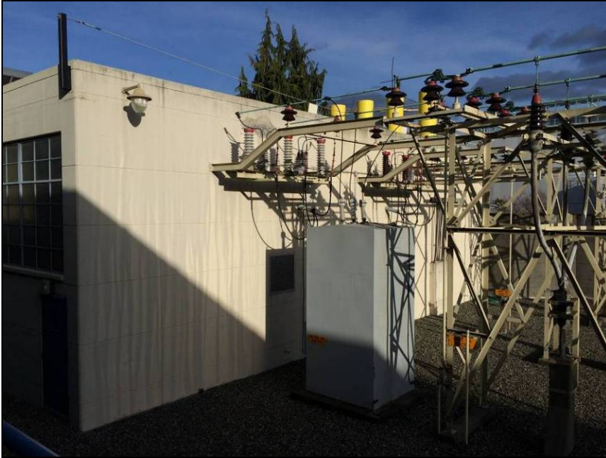
Figure 27. Above, view looking northeast at the Control Building's south facade.
